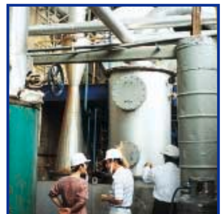
The Environmental Office and Sony Video Taiwan conduct a risk assessment exercise at the facilities of a waste treatment contractor.
