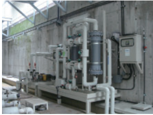
Ozone water recovery system installed at Sony Mobile Display Corporation's Yasu Plant
